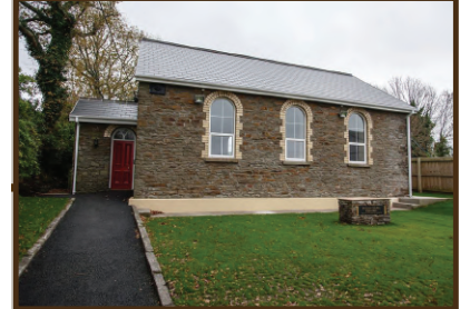
06 Pisgah Chapel is re-opened as a house of prayer for revival!
